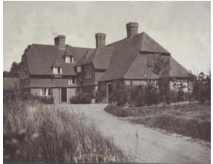
Cooper's Bridge - just occupied.
